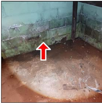
Basement walls near furnace / water heater
