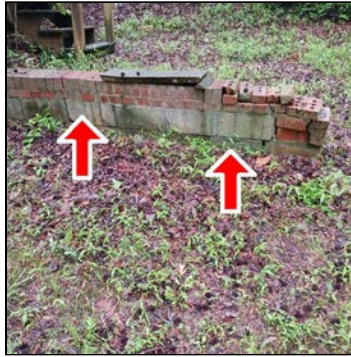
Rear retaining walls
