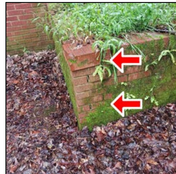
Rear retaining walls
