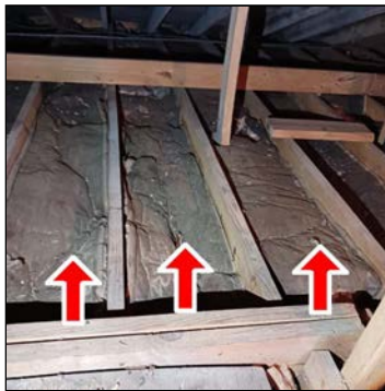
Compressed insulation in attic
