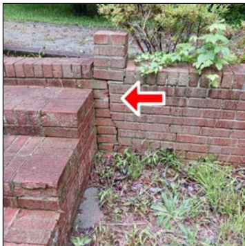
Front retaining wall
