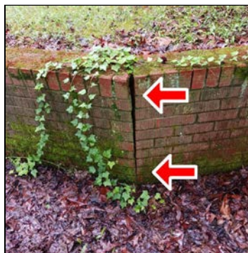
Rear retaining walls
