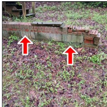
Rear retaining walls
