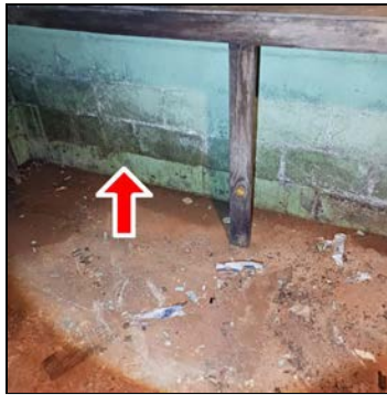
Basement walls near furnace / water heater
