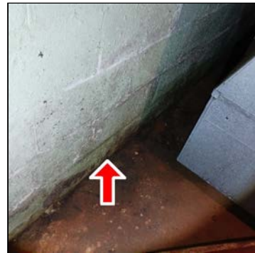
Basement walls near furnace / water heater
