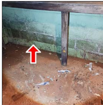
Basement walls near furnace / water heater
