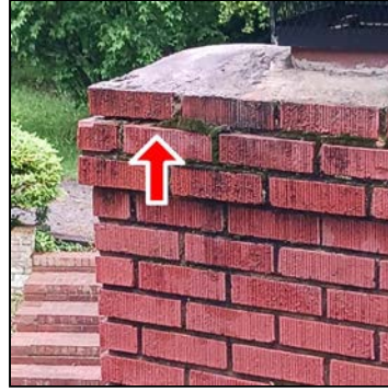
Chimney cracks
