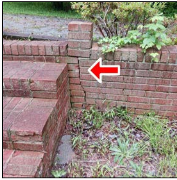
Front retaining wall
