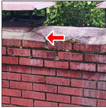
Chimney cracks
