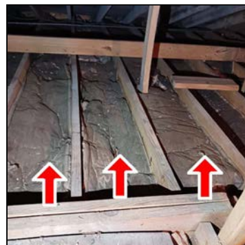
Compressed insulation in attic
