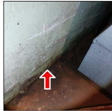
Basement walls near furnace / water heater
