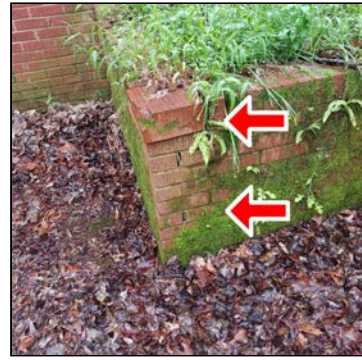
Rear retaining walls
