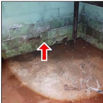
Basement walls near furnace / water heater
