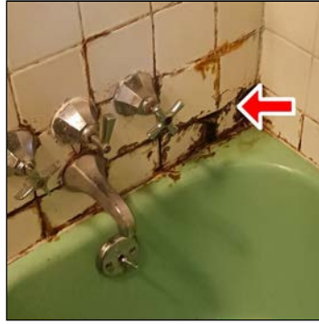
Hall bathtub tile walls
