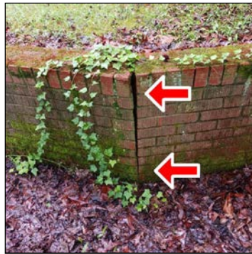
Rear retaining walls
