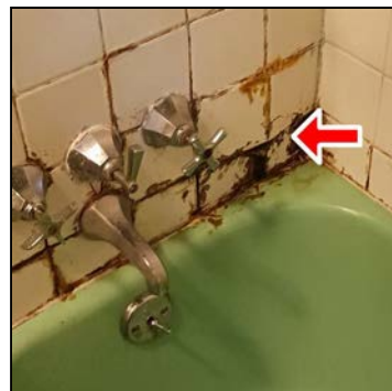
Hall bathtub tile walls
