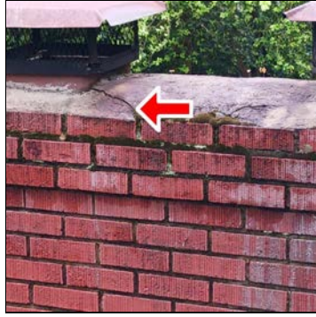
Chimney cracks
